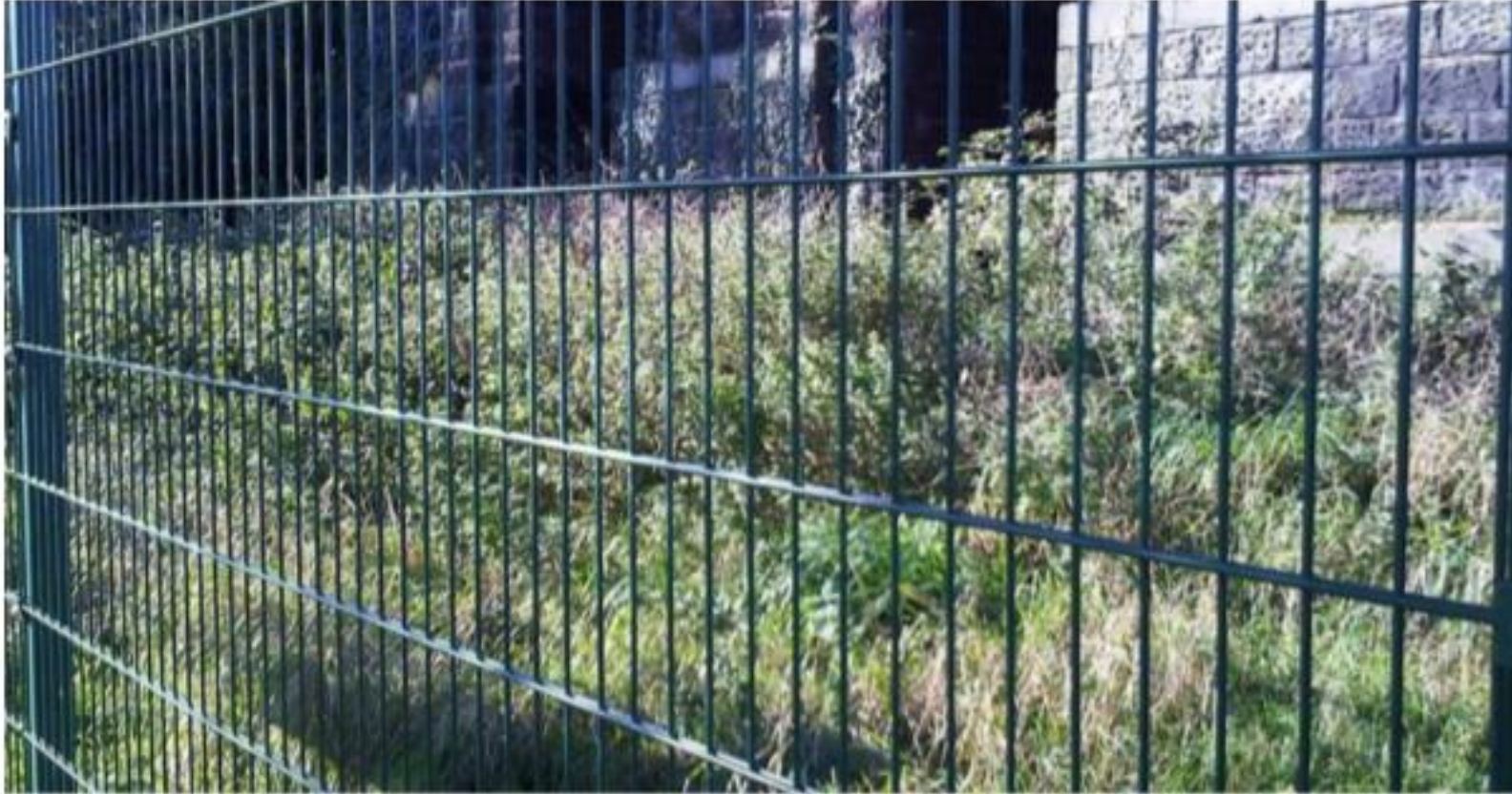
ABOVE: Proposed 2m perimeter fence, Urban Fencing DB-6 Mesh Fencing
